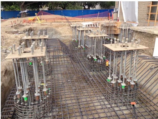
Pile cap rebar being placed at new elevators and stairway addition.
