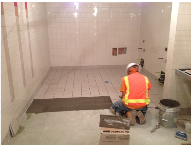
Restroom tile installation in progress.
