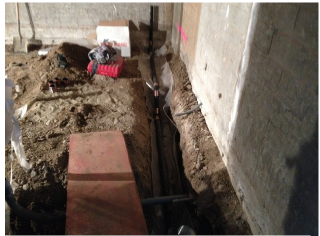
Underground plumbing activities ongoing at ground floor restrooms.
