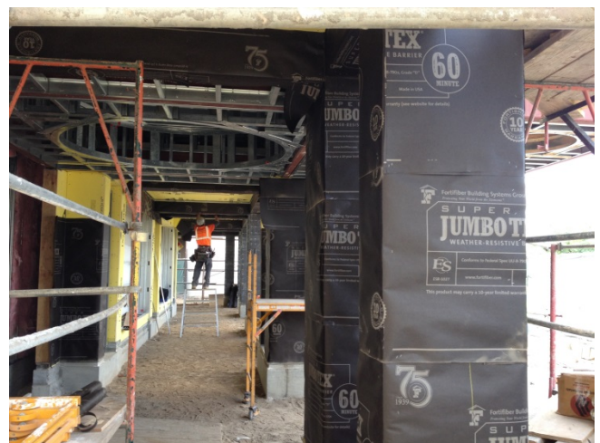
Covered walkway waterproofing and metal lath install ongoing.
