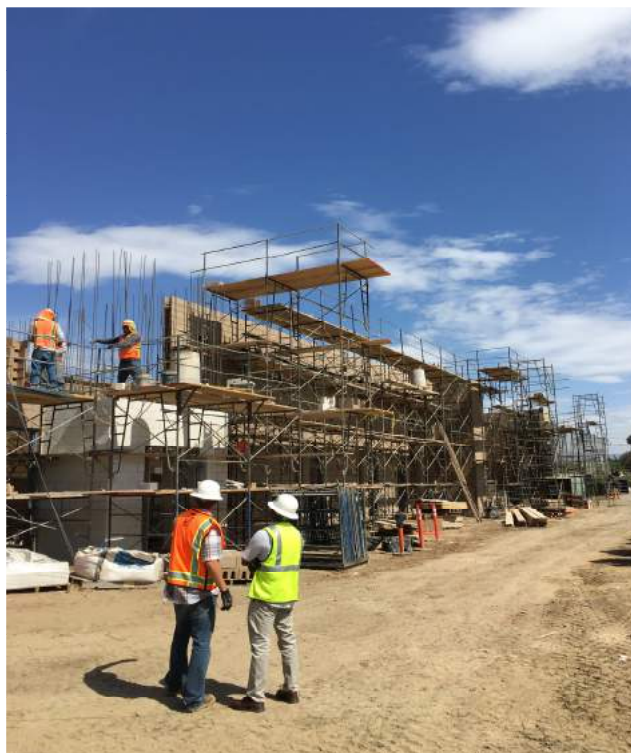
Central Plant Construction Zone
