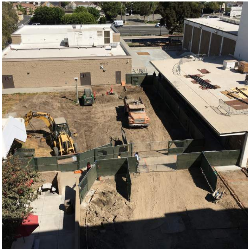
Phase 3 Construction Zone
