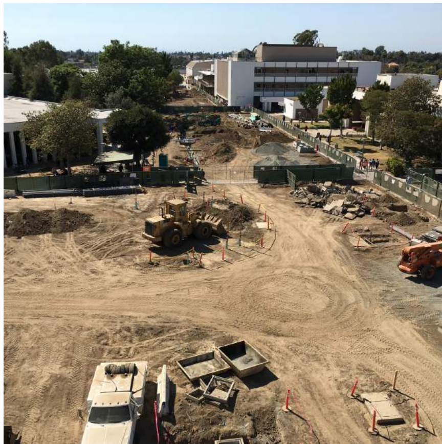
Phase 5 Construction Zone
