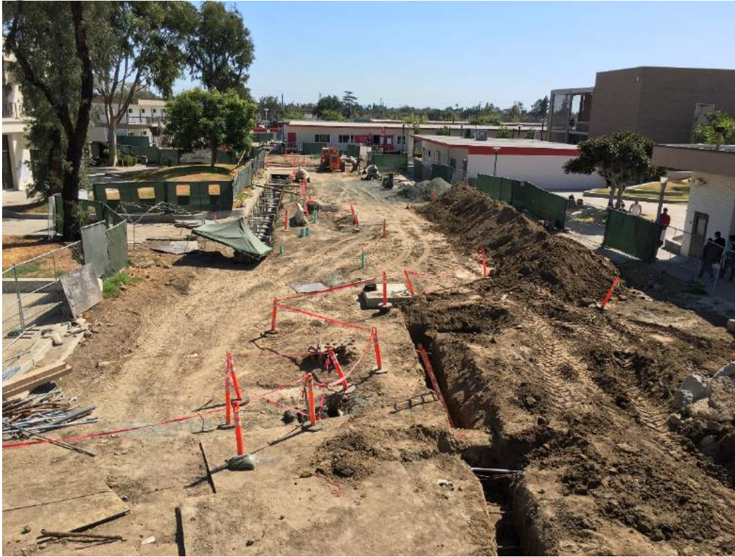
Phase 4 Construction Zone
