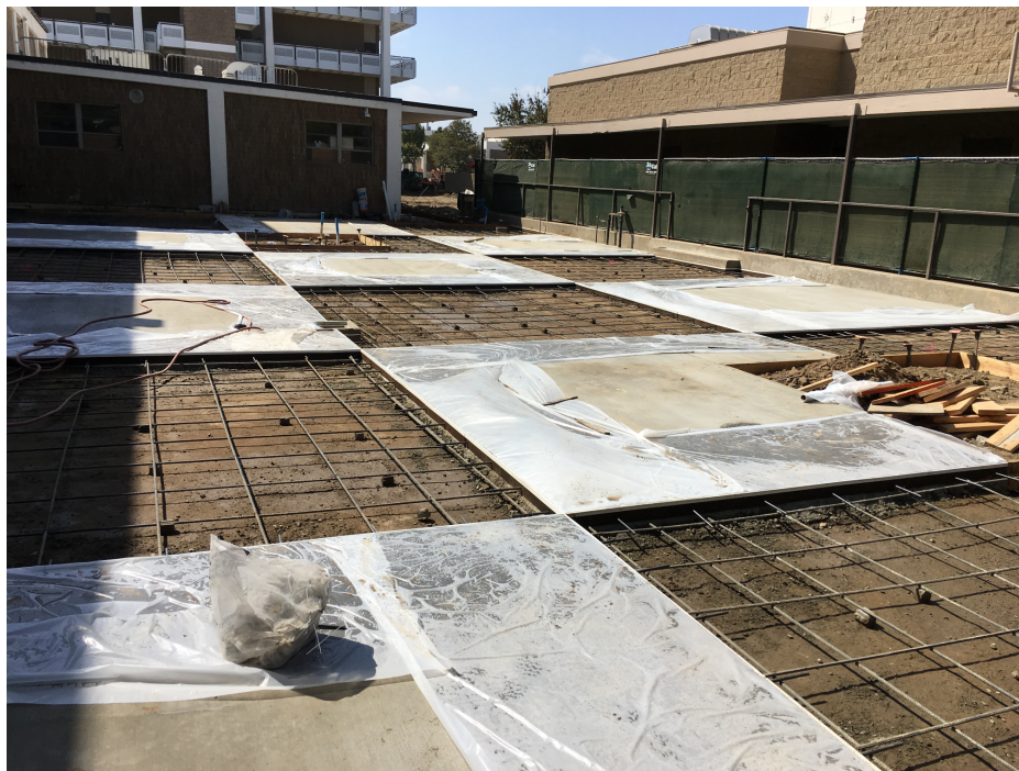
Concrete pour between Buildings N and P (Phase 3)
