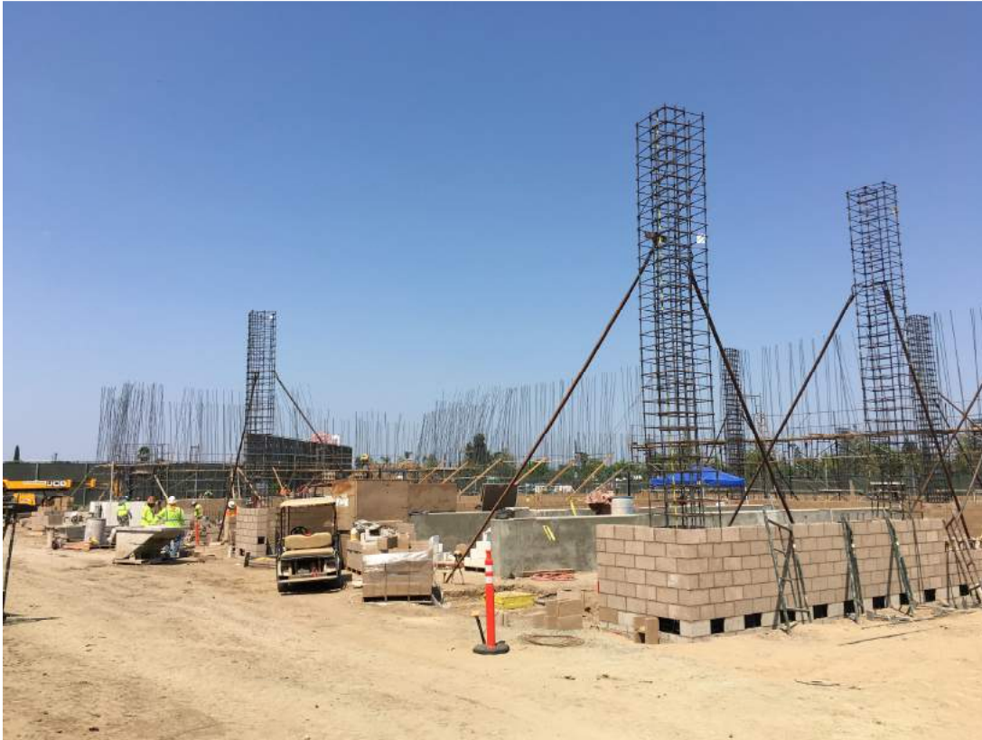
Central Plant Construction Zone
