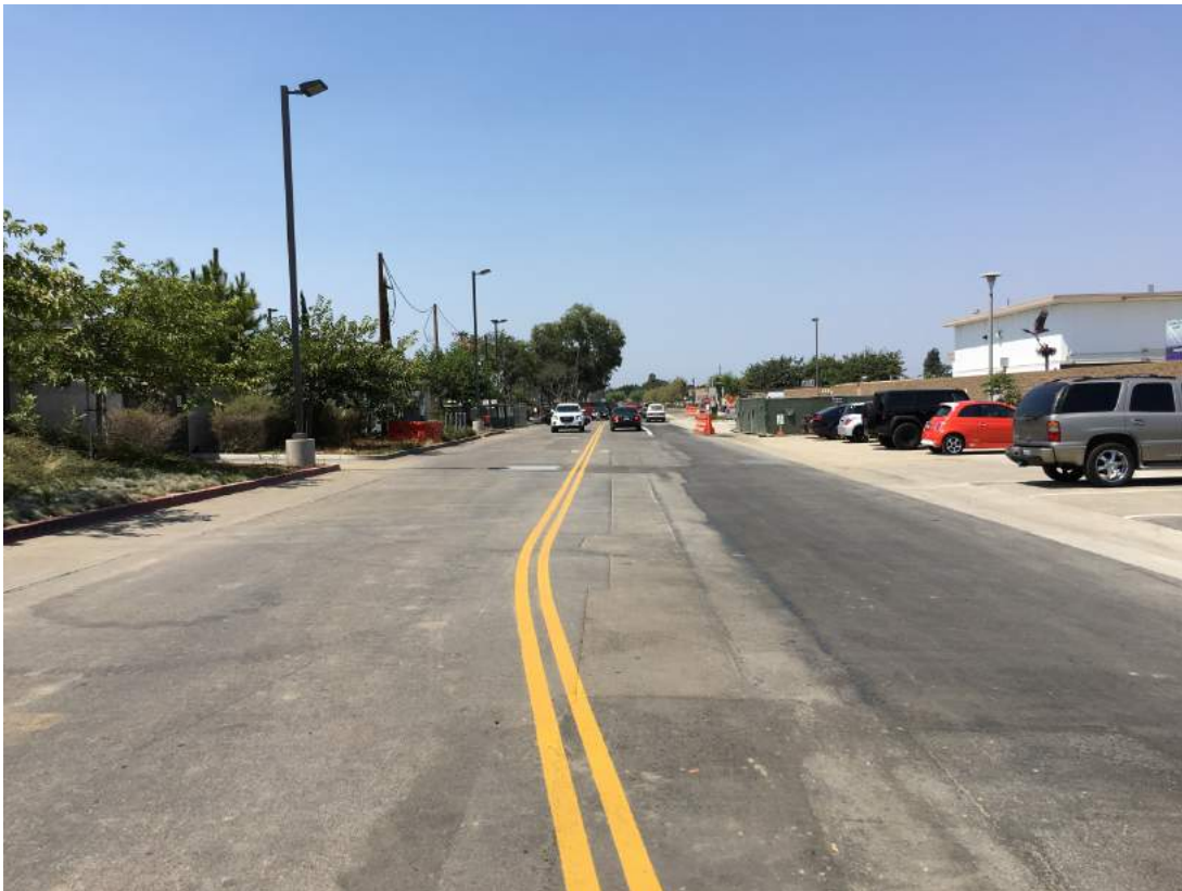
Asphalt paving and striping (Campus Road)
