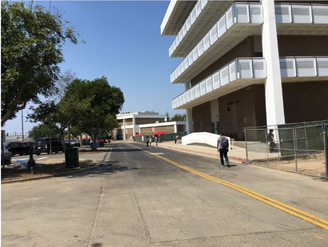
Asphalt paving and striping (Lot 6)
