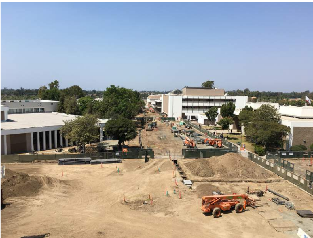
Phase 3, 4 and 5 Construction Zone
