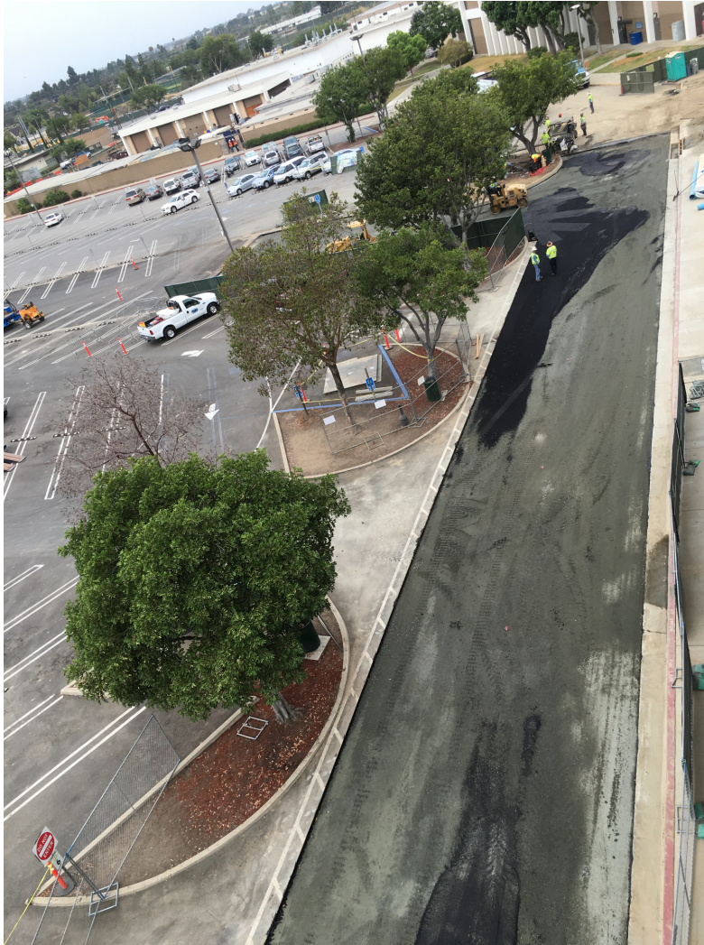
Lot 6 Asphalt Paving
