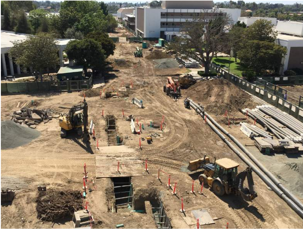
Phase 4 and 5 Construction Zone
