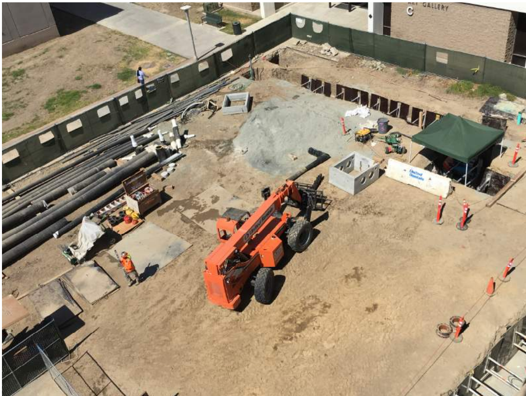
Phase 3B Construction Zone
