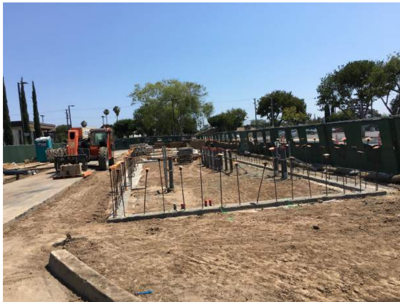
Install forms and rebar (Electrical Building)
