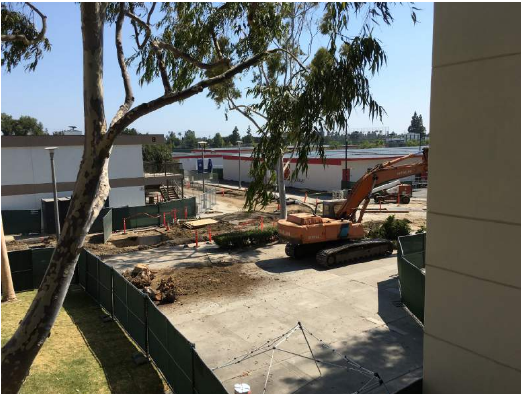
New construction fencing & small tree/shrub removal (Phase 4)
