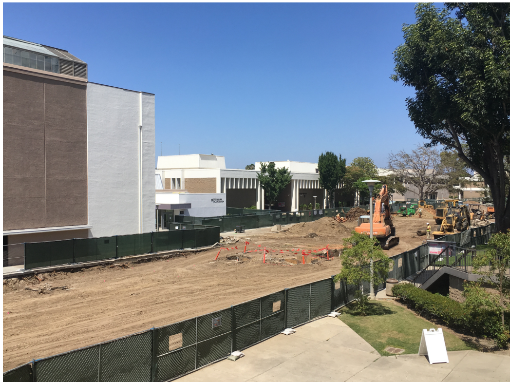
Phase 5 clearing and grubbing
