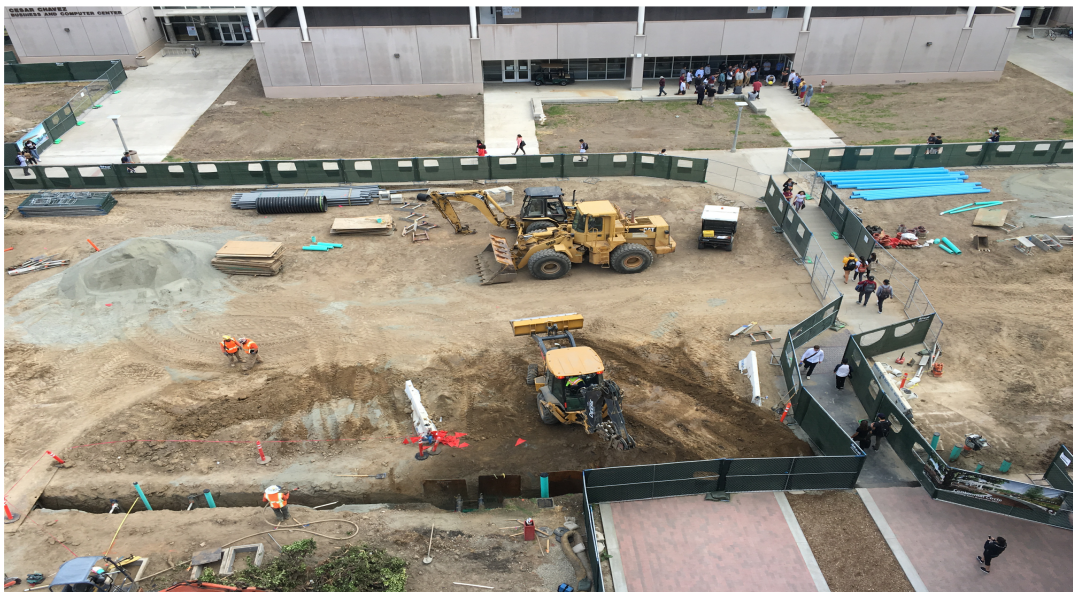
Installation of Sewer line North of Dunlap Hall (Phase 3)
