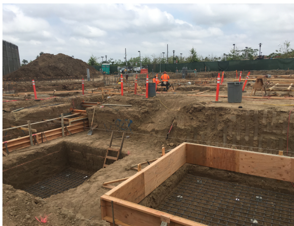
Install foundation rebar at Central Plant
