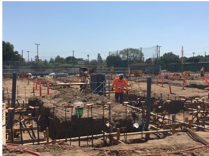
Install foundation rebar at Central Plant
