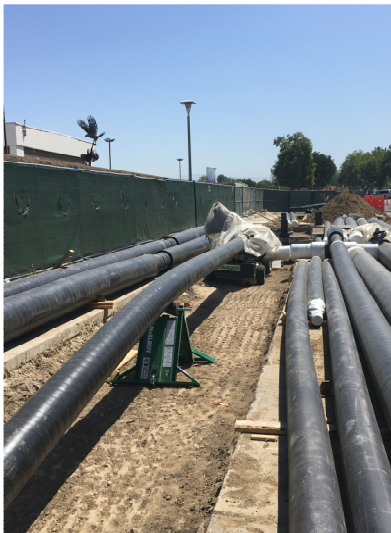
Install and test chilled water piping at Campus Road
