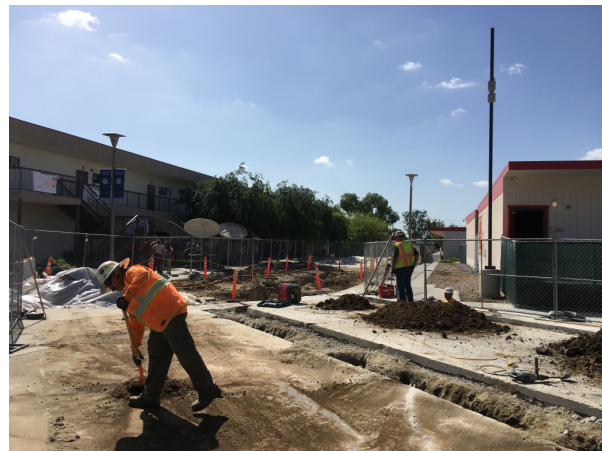
Excavate storm water and sewer at Middle College Road (Phase 2)
