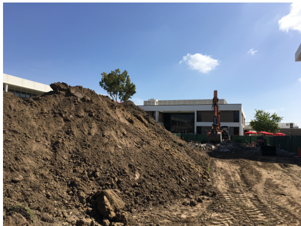
Clear, grub landscaping, demo and excavate power duct bank at Central Courtyard (Phase 3B)
