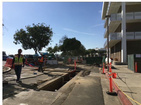
Installation of domestic water piping at Phase 2
