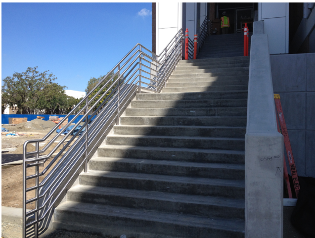
Stainless steel handrail installed at new monumental stairway.
