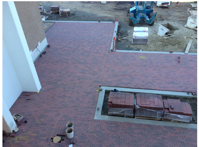
Unit pavers being installed on northwest end of Dunlap Hall.
