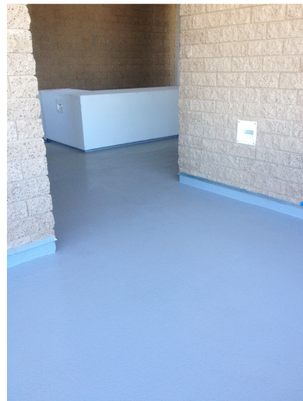
Traffic coating applied at new addition.
