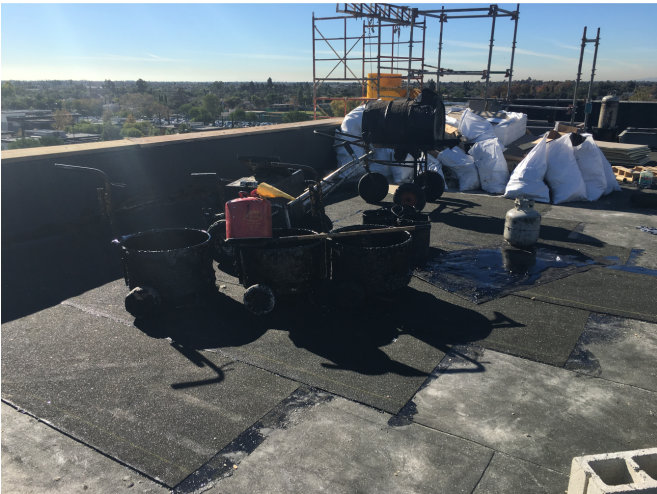
Old cellular platform has been removed and roofed area.
