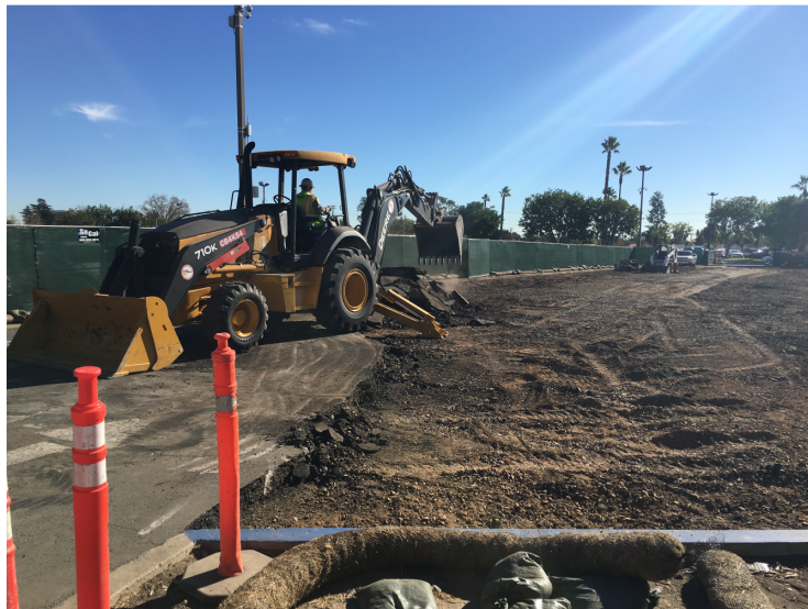
Asphalt being removed from a portion of Lot 6.
