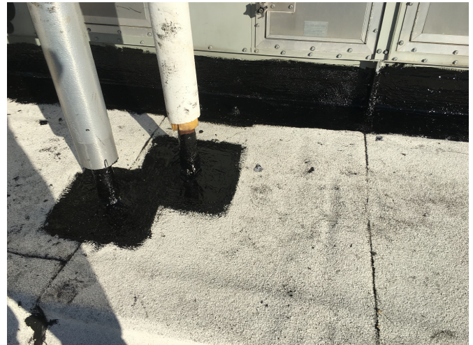
Liquid flashing applied around HVAC unit and pipe penetrations.
