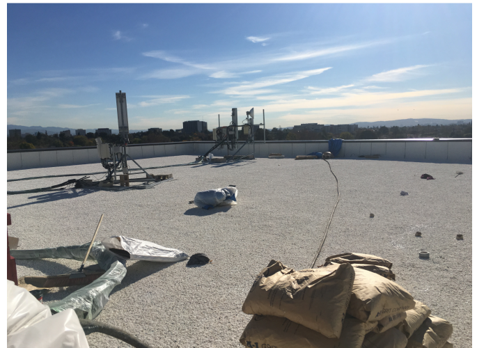
White star coating and gravel installed on Dunlap Roof.
