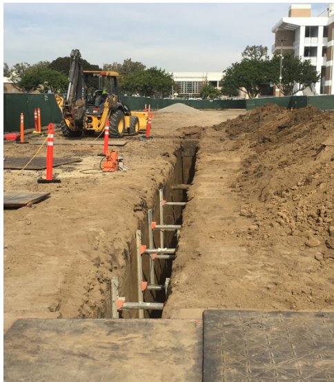
Trenching occurring in Lot 6 for underground utilities.
