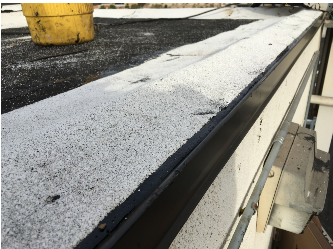
Edge metal installed on penthouse roof edge.
