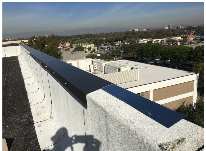
Counterflashing and coping being installed on top of parapet walls.
