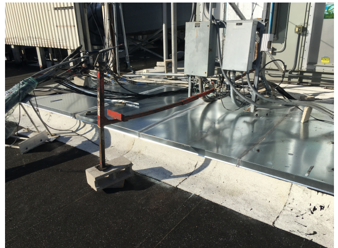
New metal pan installed over re-roofed cellular equipment platform.
