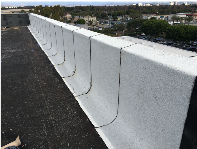
White capsheets being installed on parapet walls.
