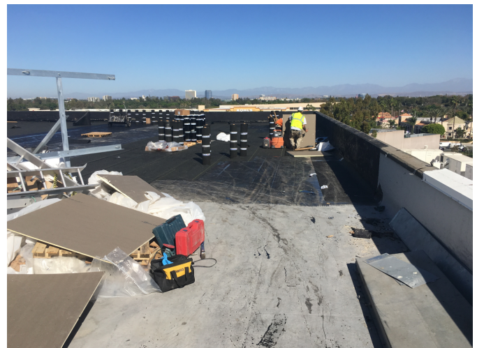
Capsheet being installed on northeast section of roof.
