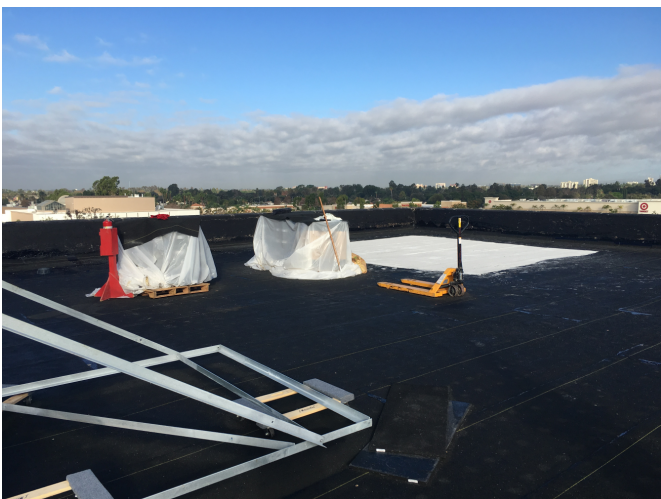
Capsheet installed on northwest section of roof with White Star and mineral coating applied to section for Sprint equipment.
