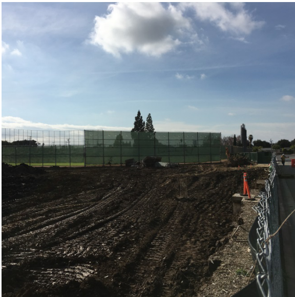
Existing Restroom Building Removed and prep for over excavation for new Bldg. pad
