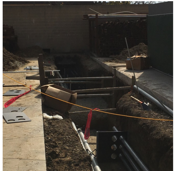
Phase 2 new electrical conduits between Building J & K
