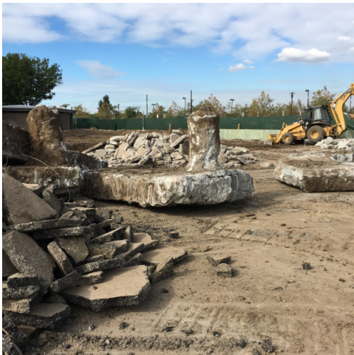
Removal of existing footings under the tennis courts at new Central Plant
