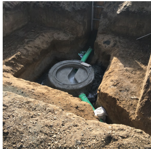
Installation of Sewer Man-Hole Bottom at Phase 1
