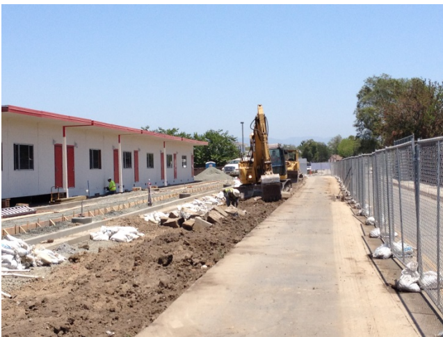
Demo operations on north lane of Campus Road.
