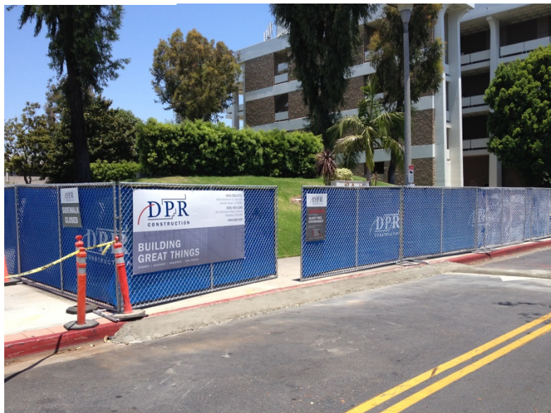
DPR construction fence around Dunlap building and amphitheater.
