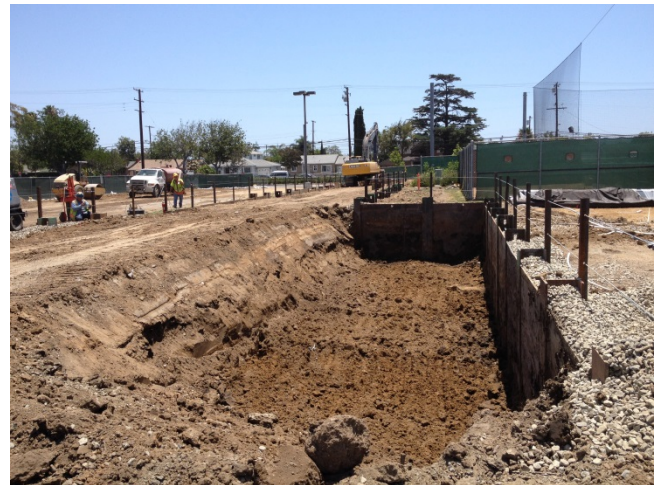
Excavation at east percolation field.
