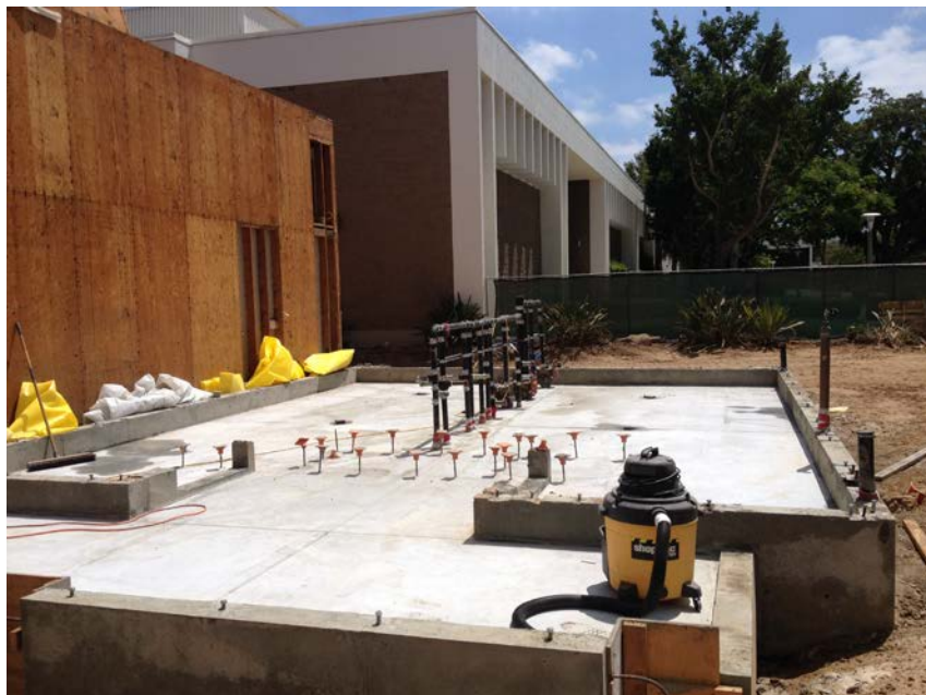
Slab poured at restroom addition, south of Planetarium.
