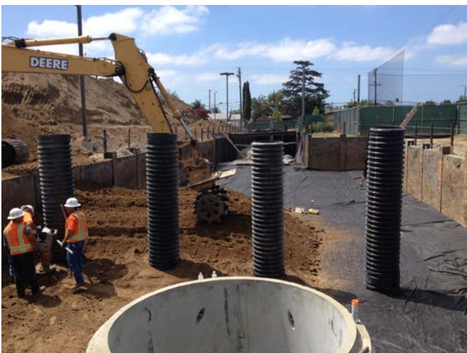
Soil being backfilled at east percolation field.
