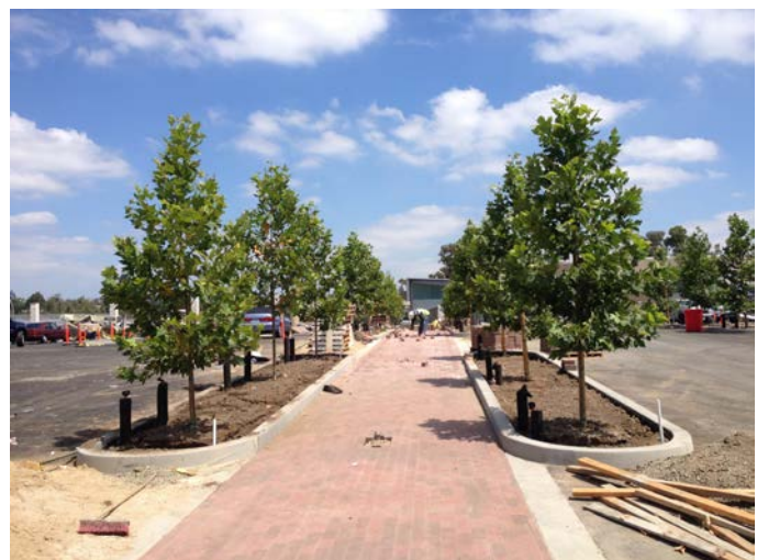
Pavers being installed at north end of pedestrian walkway. Trees installed in parking lot planters.
