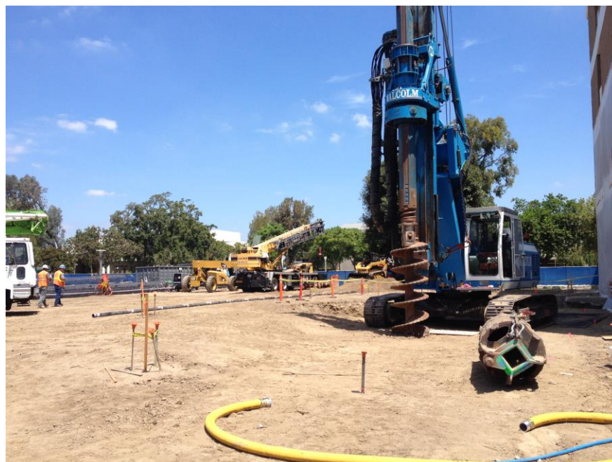
Drilling rig set up ready to start drilling piles.
