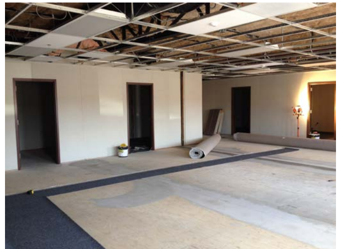
Carpet installation at future office space portables.
