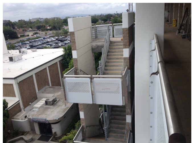
Guardrail panels being installed at stairways.
