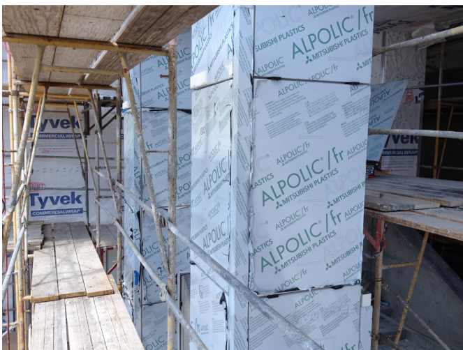
Centria panels being installed on columns at new stairway.
