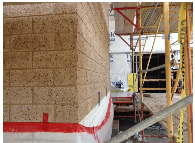
CMU veneer being installed at new addition.
