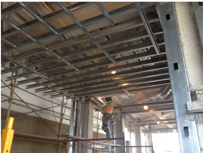
Ceiling framing being installed on 3 rd floor new addition walkway.
