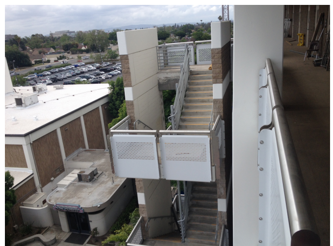
Guardrail panels being installed at stairways.
