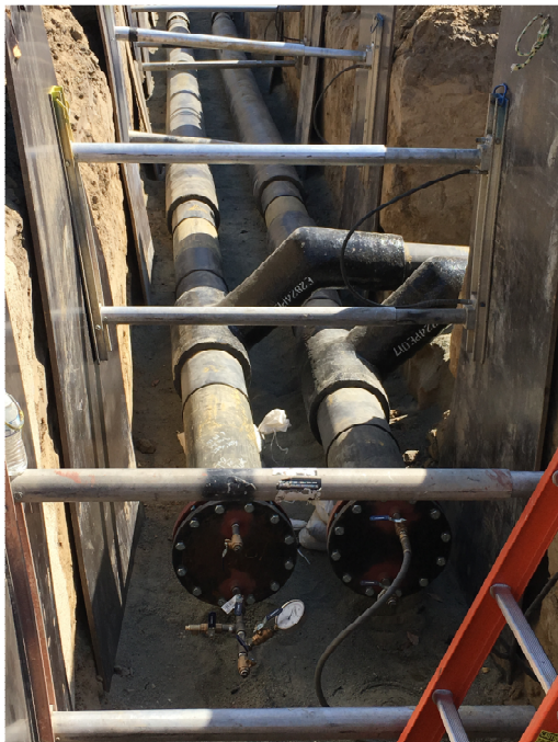
Hydronic pipe testing and inspection (Phase 1 - Lot 6)
