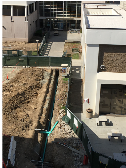
Install sewer line (Phase 3A.3)
